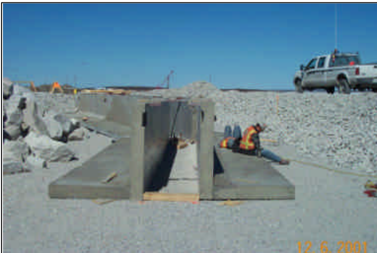
Fig. 7: Precast concrete guide wall.
