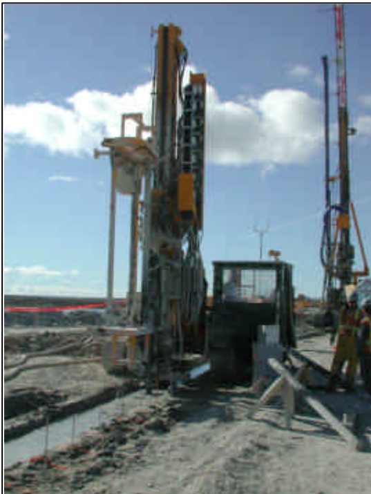
Fig. 12: UBW 09 drilling jet grout injection holes
