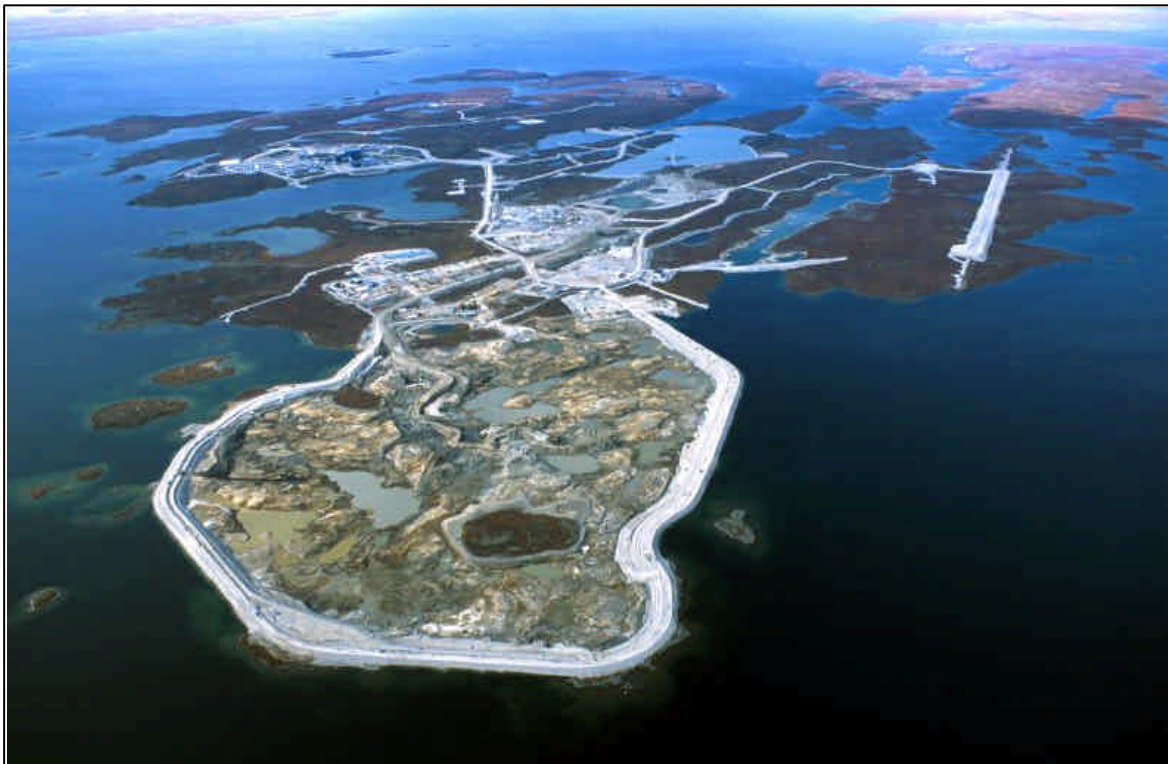
Fig. 15: Dike pool dewatered – October 2002
