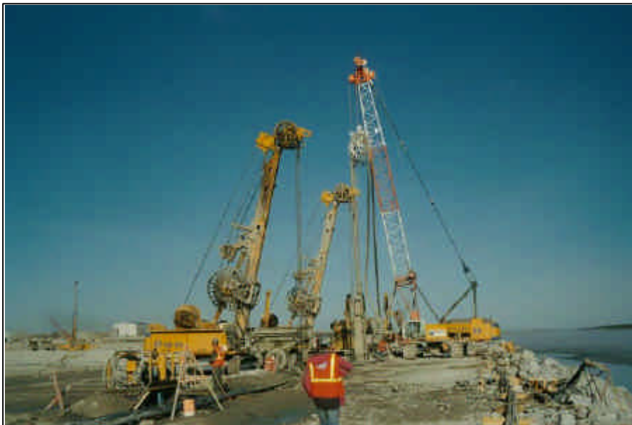
Fig. 9: Cutter and grab used in panel wall construction
