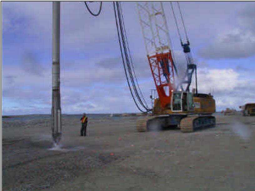
Fig. 6: Compaction with TR75 deep vibrators
