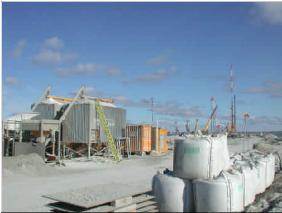
Fig. 13: Jet grout mixing and pumping station, with BG 22 in the background.
