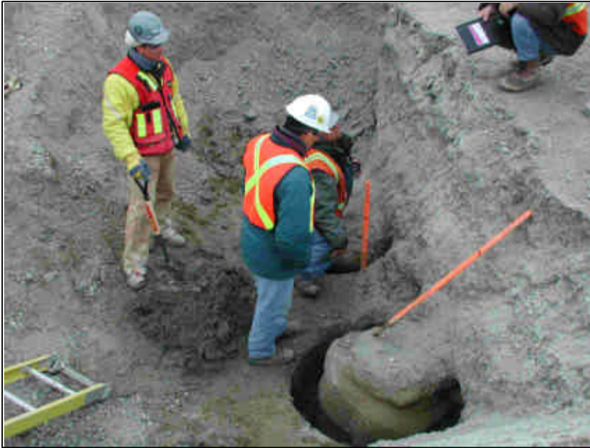
Fig.11: Excavation of test columns in frozen till
