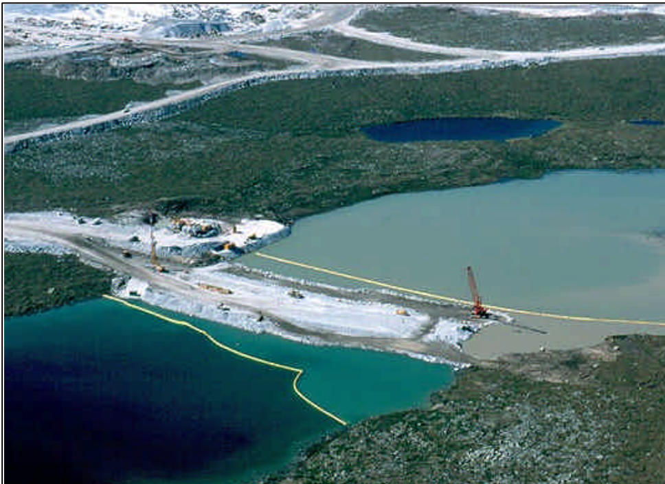
Fig.10: Jet grout injection at the North Inlet dike
