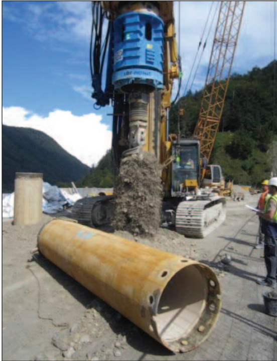
(f) Construction of the drainage piles.
