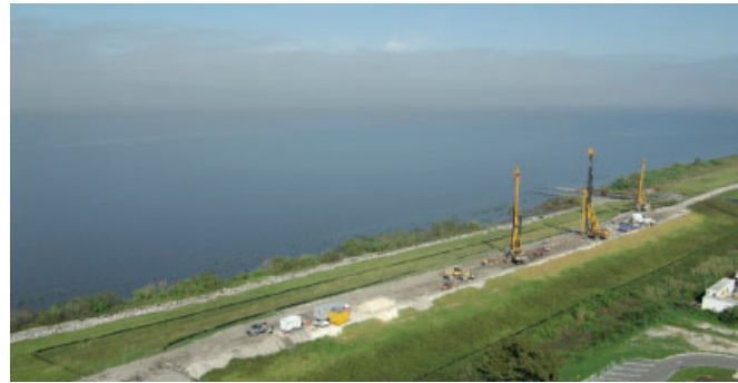
Cutter-Soil-Mixing, Herbert Hoover Dike (USA)
