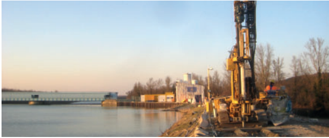
Curtain grouting, Marckolsheim (France)
