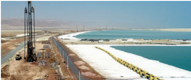
Double phase Cut-off Wall, Arab Potash, Dike A (Jordan)
