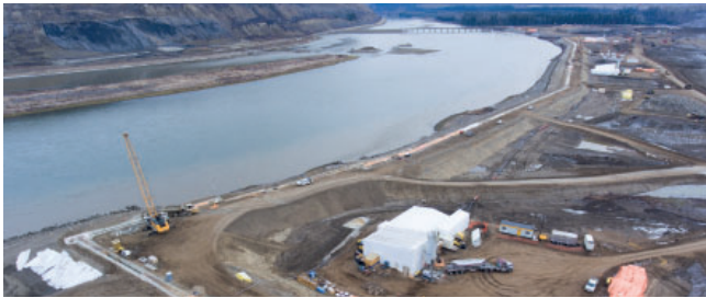
Single phase Cut-off Wall, Site C (Canada)
