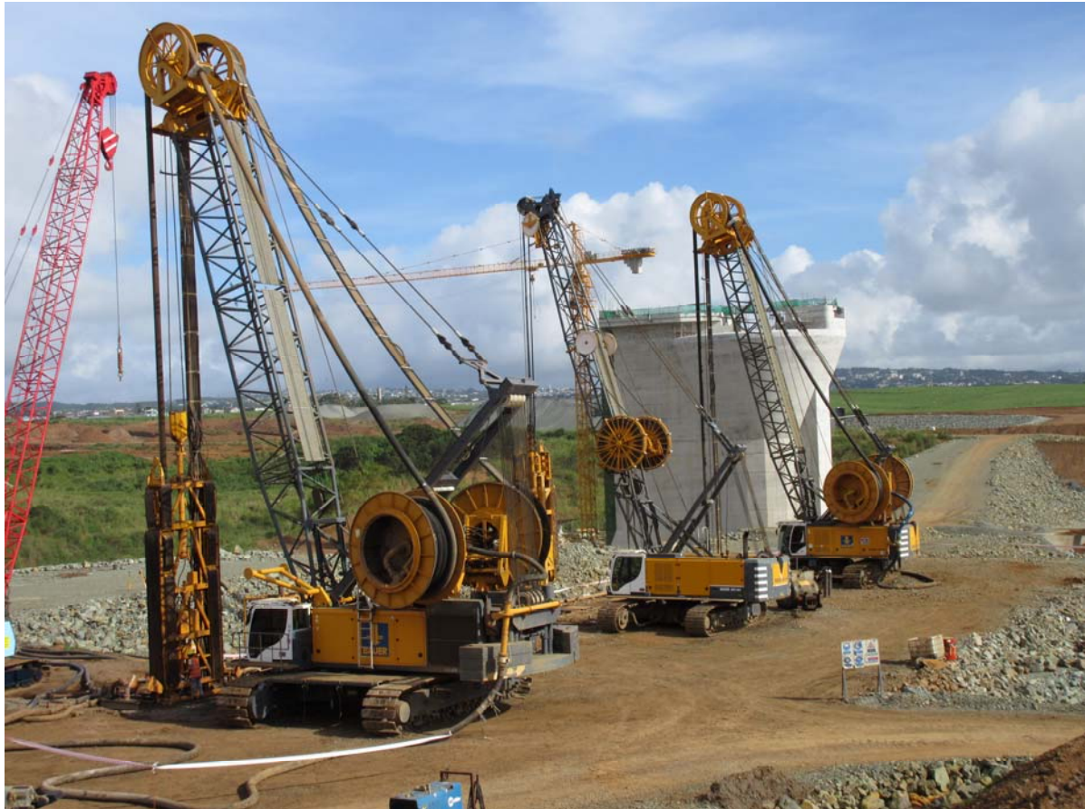
Photo 2. Permanent concrete cut-off wall excavation by Bauer Trench Cutters at Bagatelle Dam Project.
