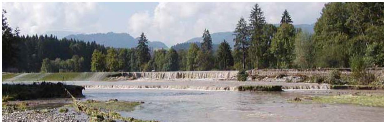
Photo 1. Levee-embankment being overtopped by flood water – MIP-cut-off wall still being in place.
