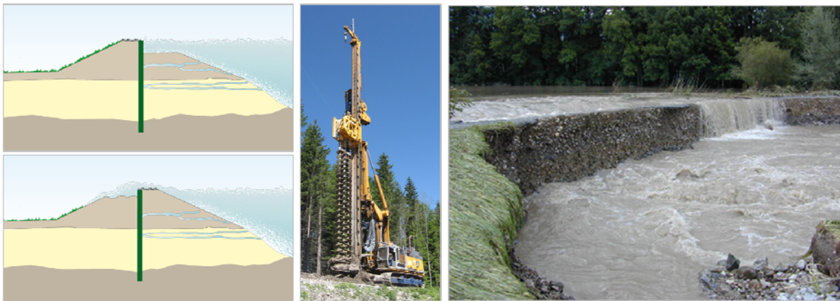
Fig. 1. Mixed-in-Place 3-auger technique. A permanent MIP-wall prevents levee to collapse during flood event. © BAUER Spezialtiefbau GmbH
