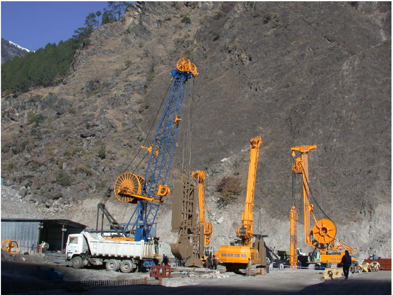
Job site set up
