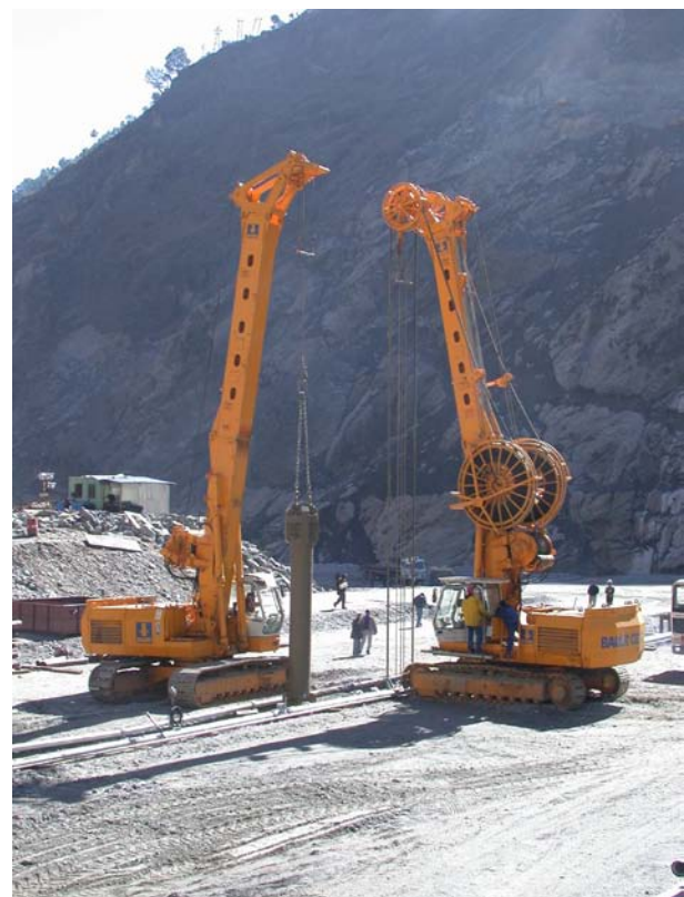
Bauer cross chisel and Bauer DHG hydraulic grab
