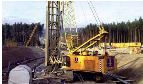
Figure 2. Trench Cutter at Brombach Main Dam, Germany 1984
