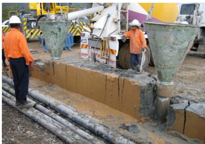
Figure 15. Up-rising cohesive plastic concrete
