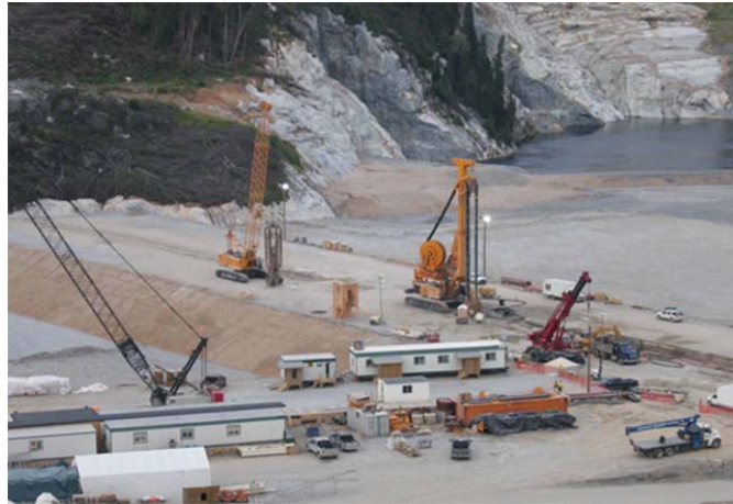
Figure 18. Set-up for cut-off wall at Peribonka dam, Canada
