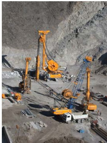
Figure 21. Site set-up for cut-off wall at Dhaulingana-1, India
