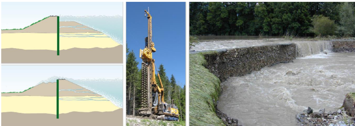
Figure 9: Mixed-in-place triple-auger technique. The MIP – wall, while being overtopped prevents levee to collapse during flood event.
