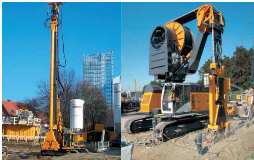
Figure 6: Kelly-guided CSM and rope suspended Tandem Side Cutter on MT 75.
