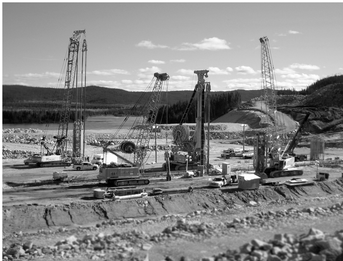
Picture 4: Two trench cutters and auxiliary equipment excavating at the main valley
