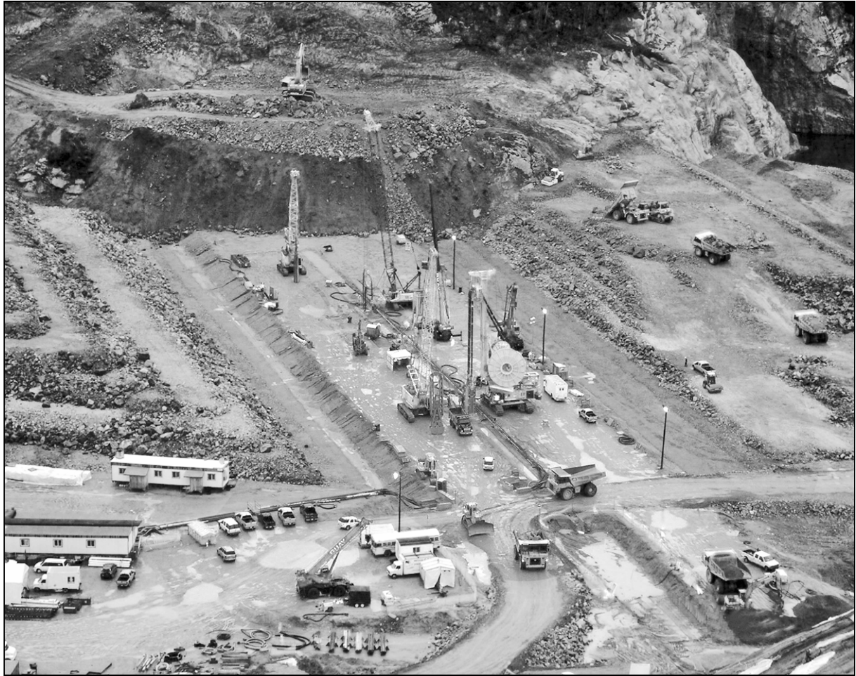
Picture 5: Cut-off wall works on the main dam
