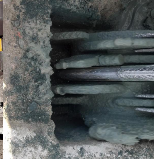
Figure 5: Rough interface created by the CSM tool overcutting a hardened panel.
