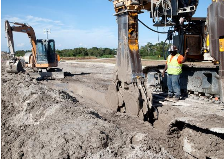
Figure 4: CSM tool BCM 5 being positioned over the pre-excavation trench.
