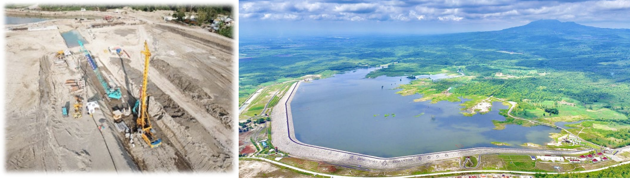
Fig. 2. Execution of secant pile wall (left), and picture showing the current status of the project
