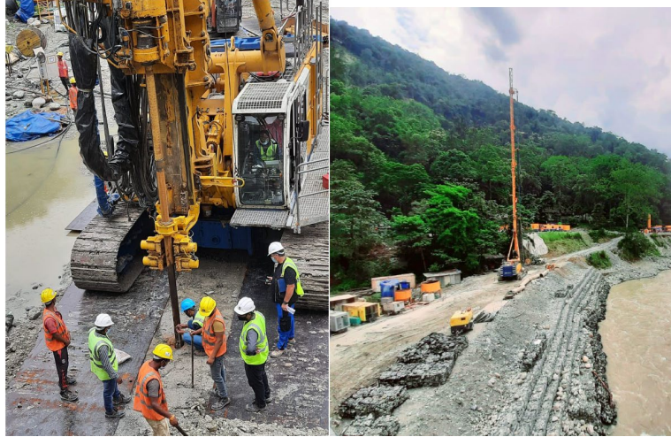
Fig. 6. Redrilling for jet grouting and predrilling of the holes in the boulder strata along the alignment
