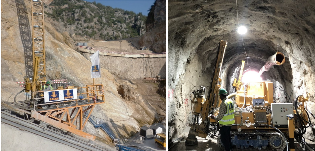
Fig. 12 Mobile platforms on special rails for drilling and grouting works on slopes, exposed bulkhead in the background (left) [1], and working in galleries using electrical drilling rig (right)
