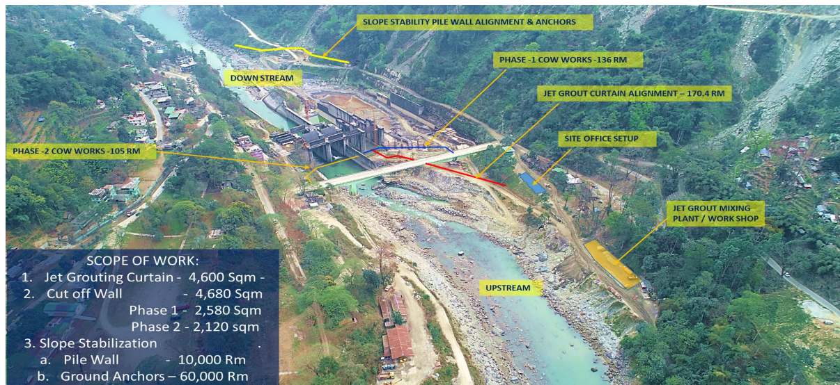
Fig. 3. Overview showing the scope of works consisting of several construction methods
